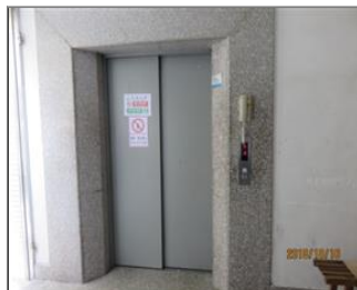
Photo of the inside of the main production hall cargo lift.JPG
