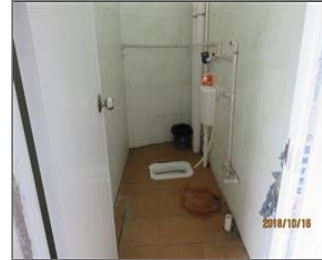
Photo of the sanitary facilities toilet.JPG
