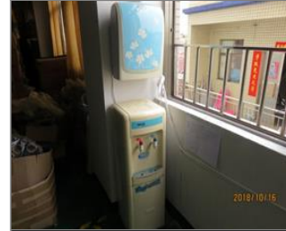
Photo of the sanitary facilities drinking water.JPG
